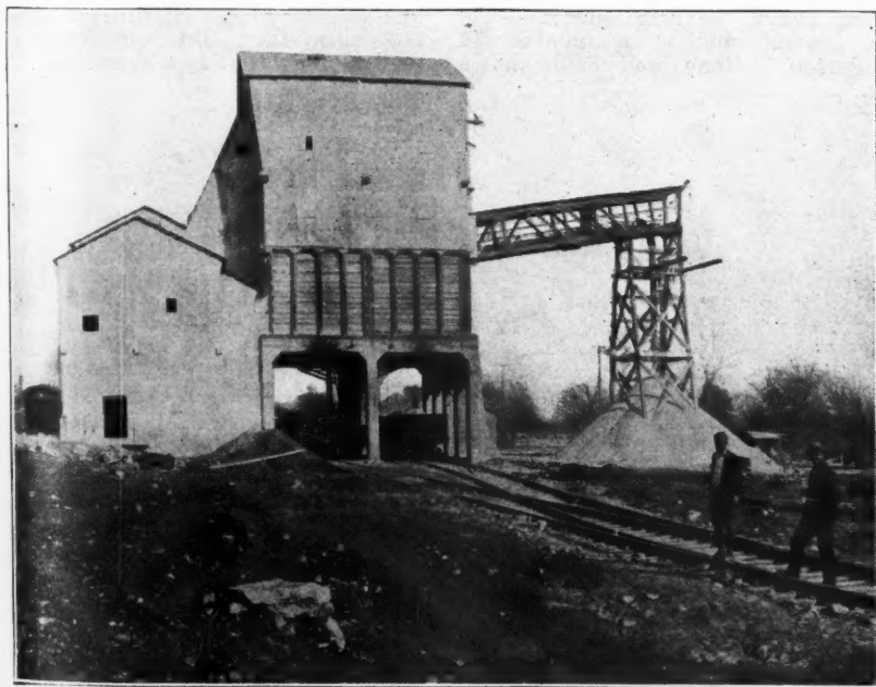
Storage Bins and Tracks
